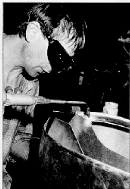
23: Pete welds the tunnel into place.
