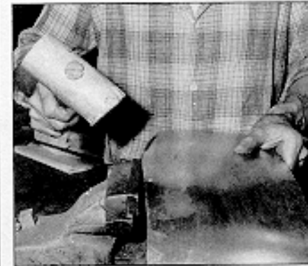
7: A double curvature is formed along the edges of the tank top.
