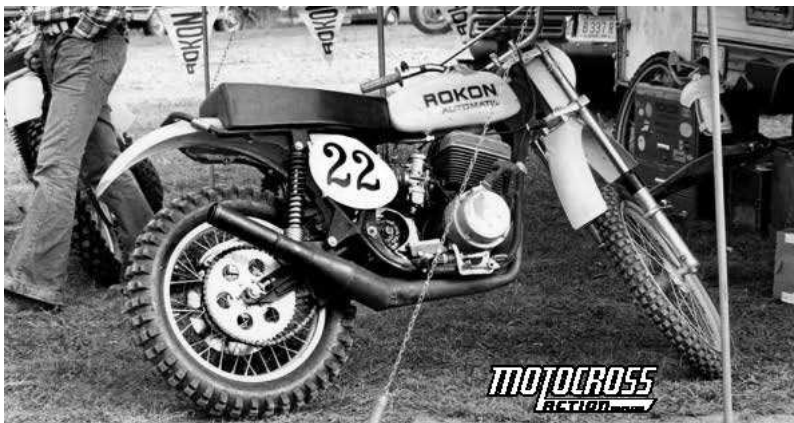
Rokon used a snowmobile engine to power the 340 Cobra. The Rokon had disc brakes, front and rear, in 1976.
